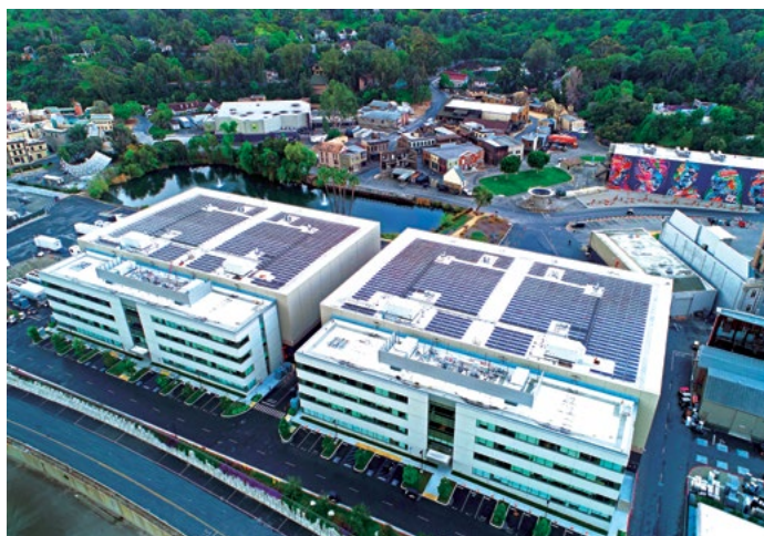
A view of the nearly 1,400 solar panels on the roofs of four sound stages at the Universal Studios Lot in Los Angeles.
